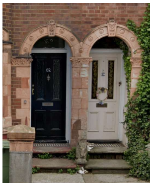
Recessed entrance with tiles
