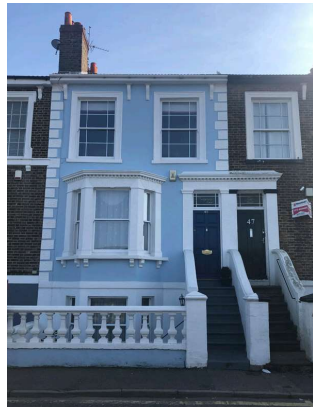
Decorative brackets under eaves
